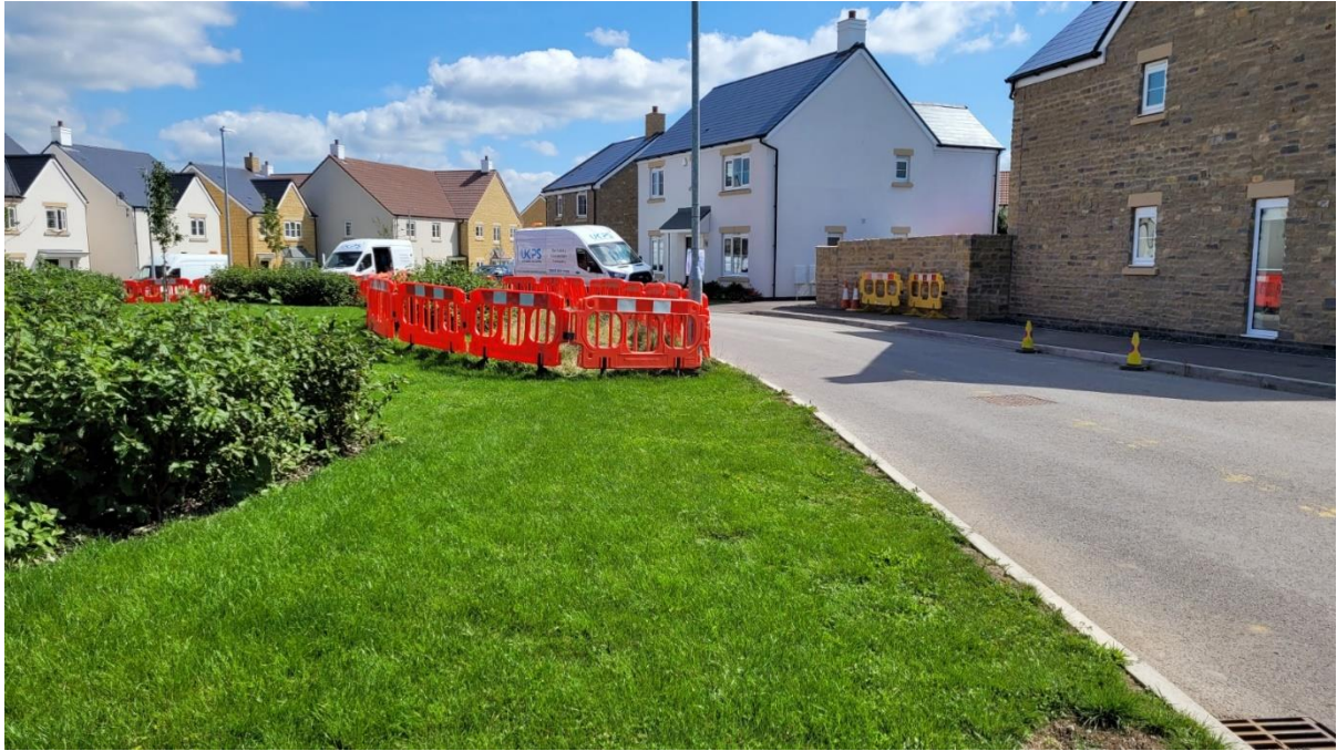
Excavation on front green
